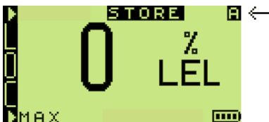
Fig. 3-34 Alarm Enabled Identifier
